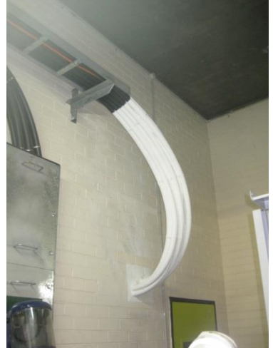
KBS Panel Seal Installation
