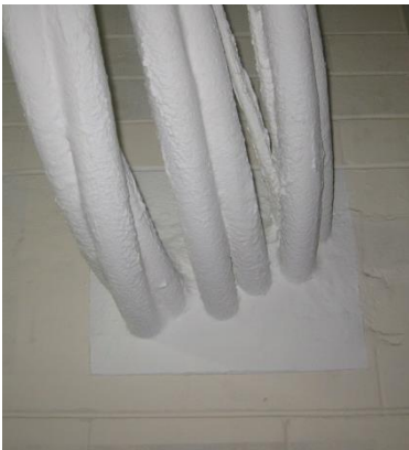
KBS Panel Seal Installation
