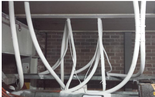
KBS Cable Coating in basement
